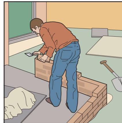
Next, the installer will construct the dwarf wall if required.
