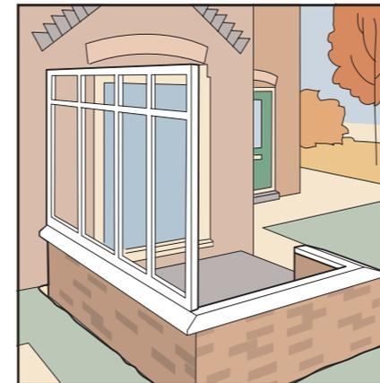
With the base in position and the dwarf walls completed, the frames making up the conservatory sides are put in place.
